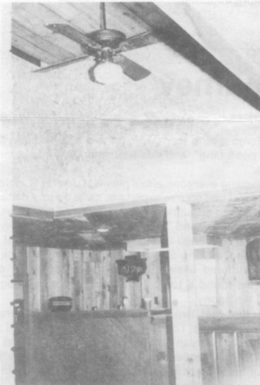
New ceiling and fan placed over the game room.
